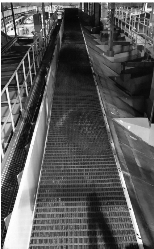
Dallas Bulk Mail Center (BMC) dangerous conditions
